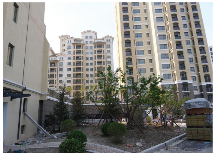
Figure 5. Residential buildings were elevated on a parking deck, separating community open spaces from the urban context.
